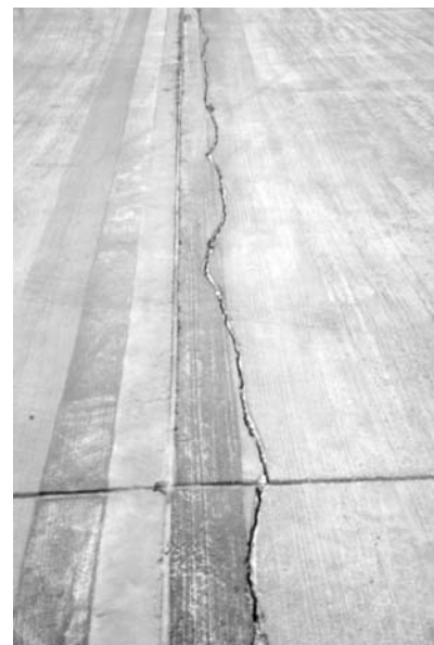
◀ Crack parallel to joint. Open 1/4". No spalling.
