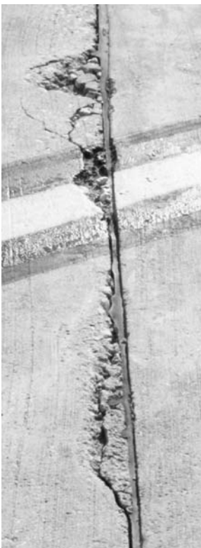
◀ Spalling along a joint.
