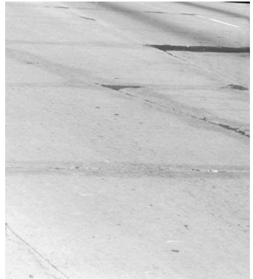
Surface discoloration near joints and cracks indicates D-cracking and severe slab deterioration.
