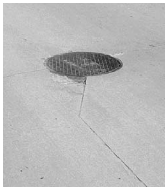
▲ Isolated spall at manhole.
