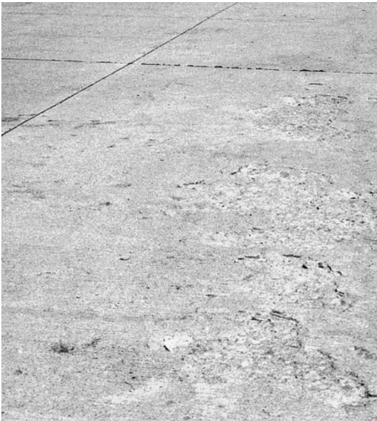
▲ Isolated spall at manhole.
