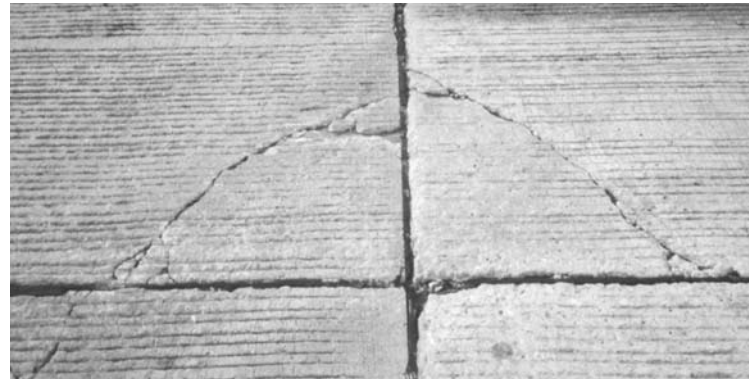
Corner cracking with slight spalling.
