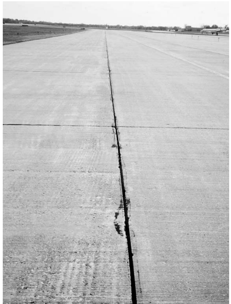
▲ Joint sealant deterioration on apron. Slab is in good condition.
