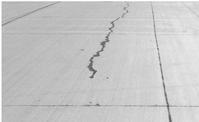
▲ Map cracking, but pavement is sound.
