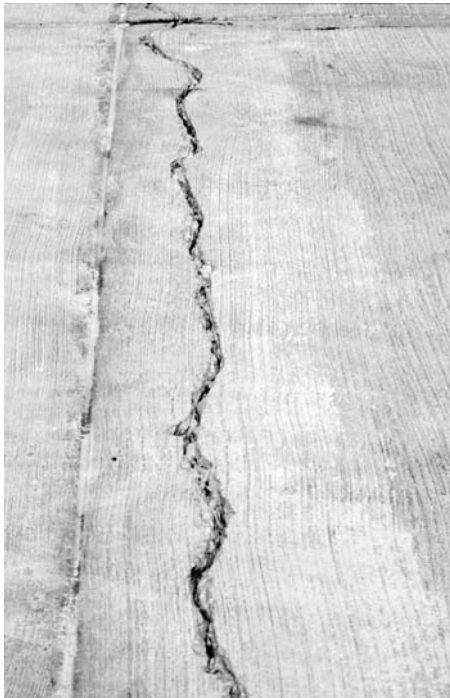
◀ Crack next to joint often caused by late sawing. Crack shows early signs of spalling.
