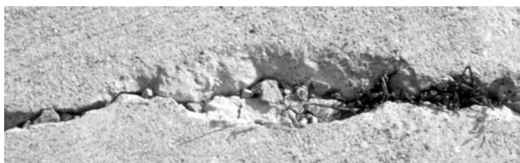
◀ Spalling along a joint.
