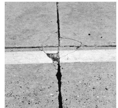
Corner cracking in all four slabs.
