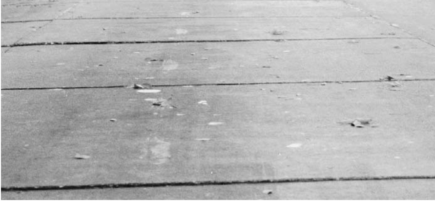
▲ Faulting of joints. Aggravated by heavy traffic in one direction. Could improve surface by grinding.
