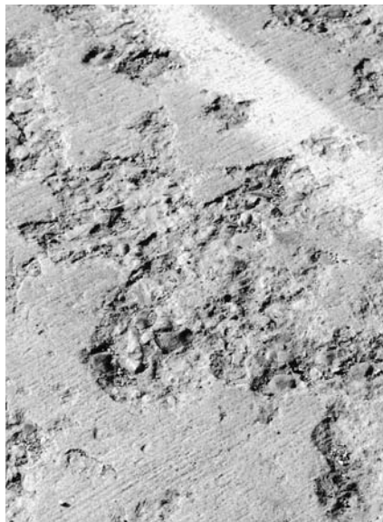
◀ Severe scaling. Some larger aggregate is loose.
