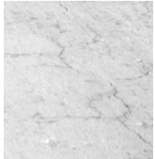
▲ Map cracking, but pavement is sound.
