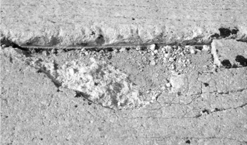
▲ Failed joint with severe spalling and pothole.
