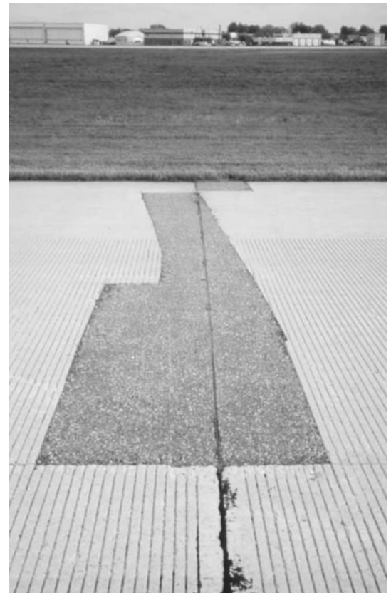
▲ Full depth joint repair. Very good condition.
